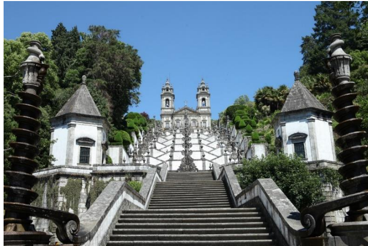
Figure 1. Sanctuary of Bom Jesus do Monte: Stairway
