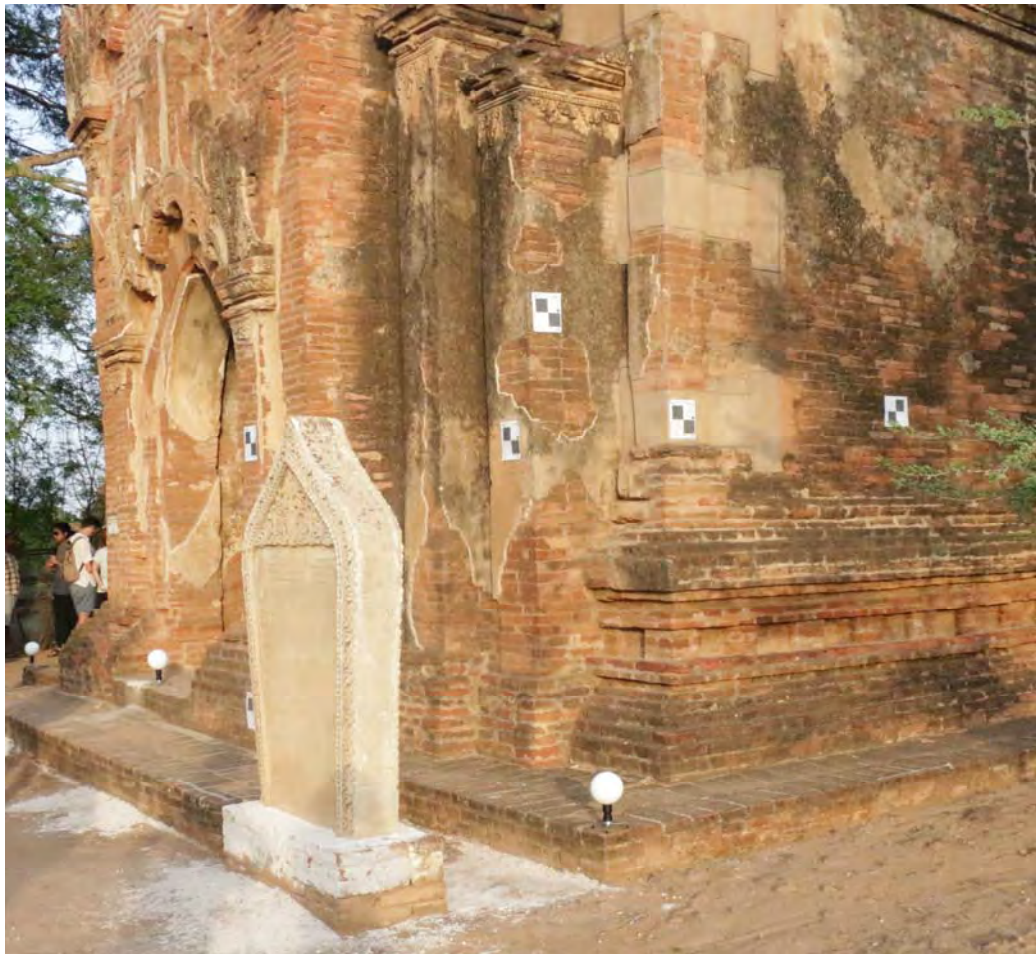
Figure 30 Image illustrating targets and sphere used to document Loka-hteik-pan temple. Image source: Author.
