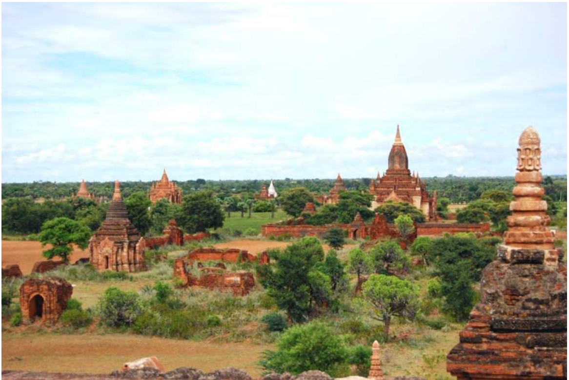
Figure 26 View of Bagan plain depicting the state of degrade affecting many of its historic built structures. Image source: Author.
