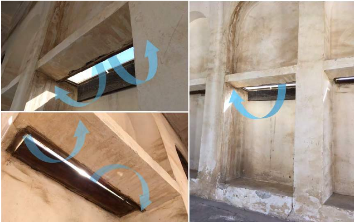
Figure 9 Example of badqeer , system. Shaikh Isa bin Ali House in Muharraaq, Bahrain. Image source: Author.
