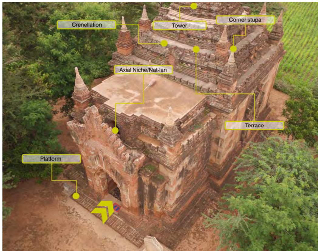
Figure 48 Description of some elements of the Loka-hteik-pan temple. Image source: Author.
