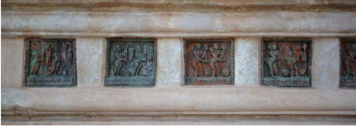
Figure 50 Ananda temple. Example of glazed ceramic tiles that decorate the high base moldings.
