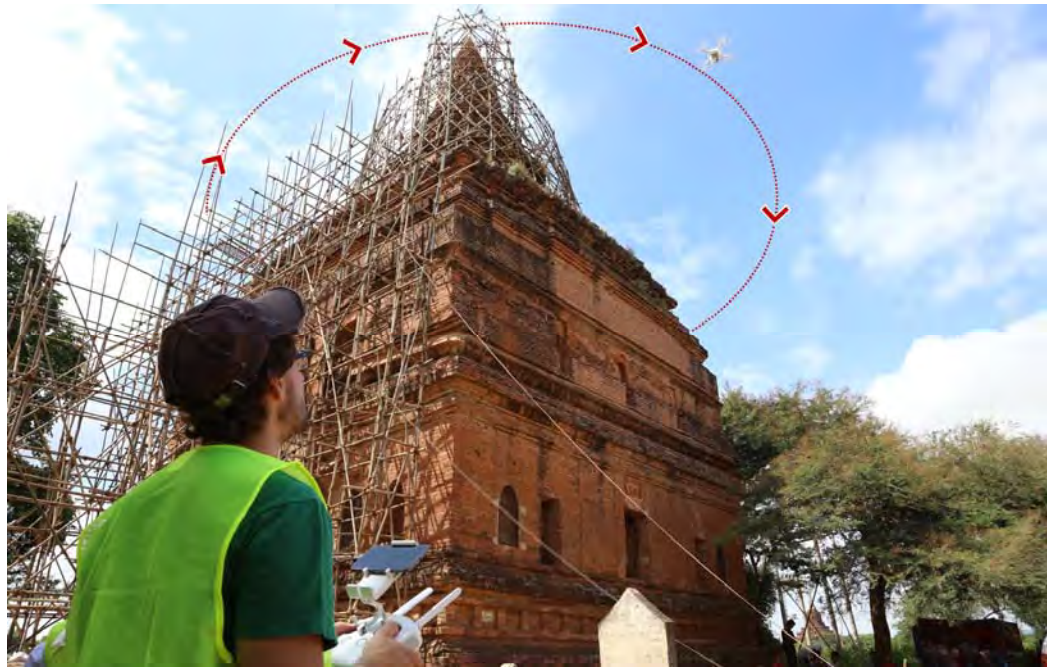
Figure 21 Example of drone flying in a pre-set circular path. Image taken by Ross Davidson and edited by the Author.
