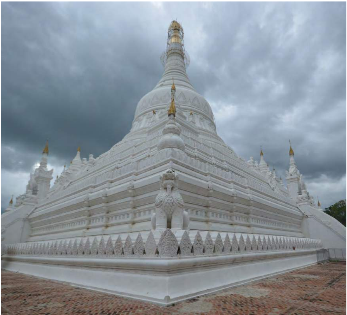
Figure 29 Example of stupa coated in stucco and whitewashed, Sandar Muni Pagoda, Amarapura (Mandalay region). Image source: Author.
