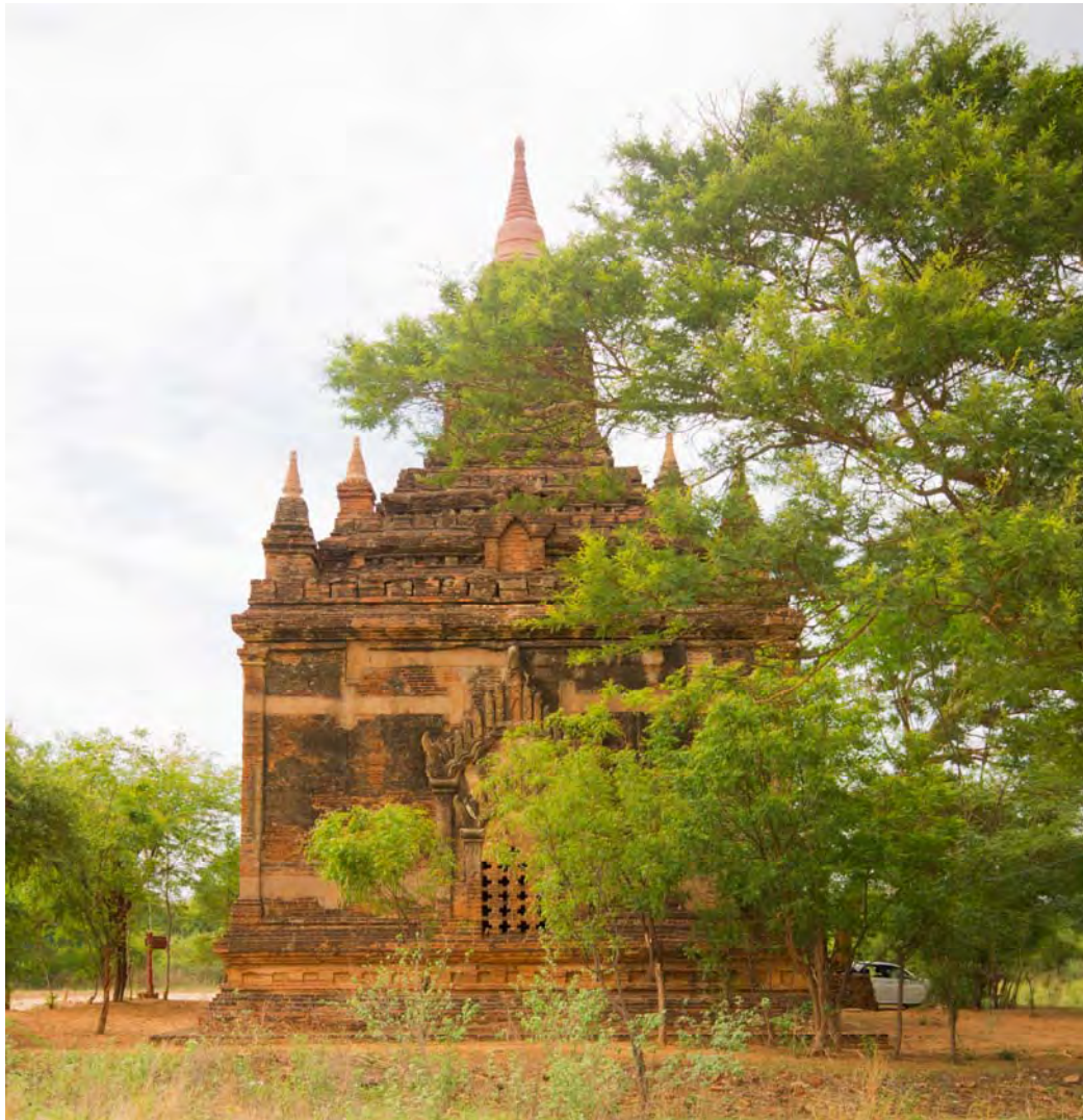
Figure 1 Loka-hteik-pan temple, south façade. Image source: Author.
