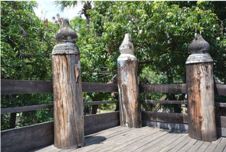
Figure 10 Wooden elements combined with stones to decrease the moisture effects. Example of the construction solutions developed to preserve the monastery structure from the heavy rain during the
