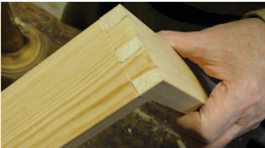
Plate 1 An example of a dovetail joint. Photo: Milo Marsfeldt Skovfoged, 2018.
